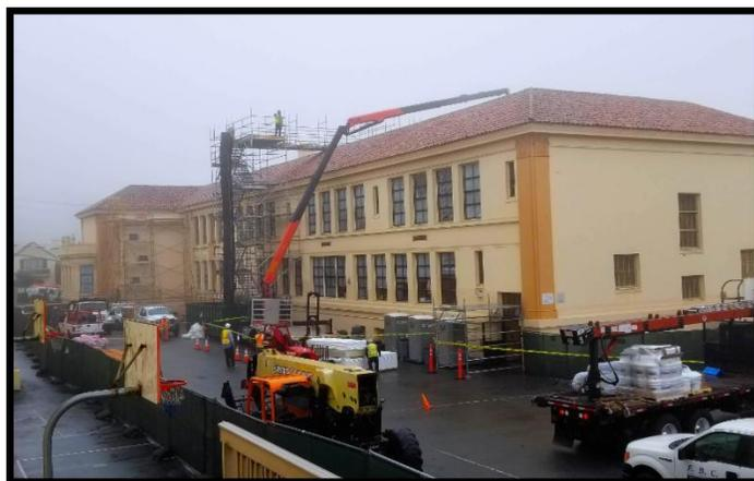
With the beginning of Summer 2018 came the beginning of Phase I of our seismic retrofit. Major work has been underway to secure the interior walls of the southern end of the school building. This southern end is the original school building and was constructed in 1930 using hollow clay tile walls. The seismic study revealed that these hollow clay tile walls would not be safe in the event of a major, local earthquake. Therefore, the walls in these rooms have either being replaced or reinforced to
